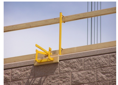
PARAPET GUARD RAIL #12090
