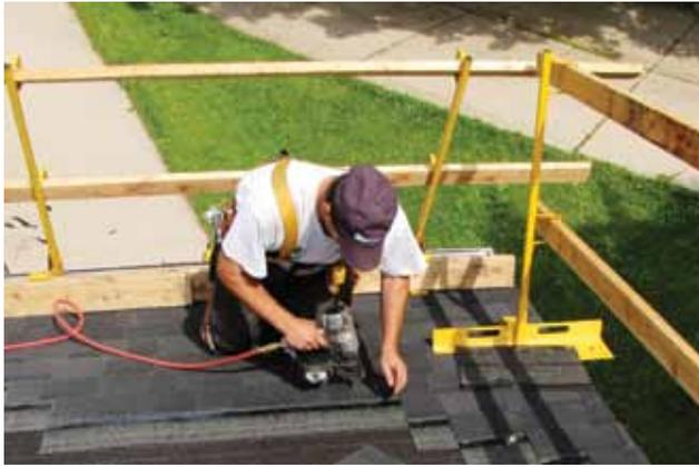
Acro Building Systems' modular guardrail system utilizes reusable components to create a simple passive fall protection solution for many different situations.
