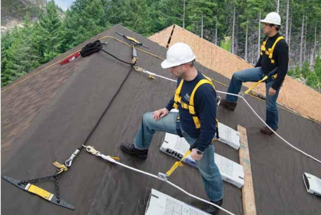
Capital Safety's Sayline horizontal lifeline system enables two roofers to work an entire roof safely and hassle-free, with complete freedom of movement.
